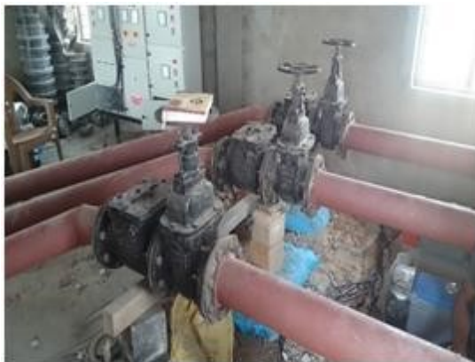
Construction pump house under construction pipe works
